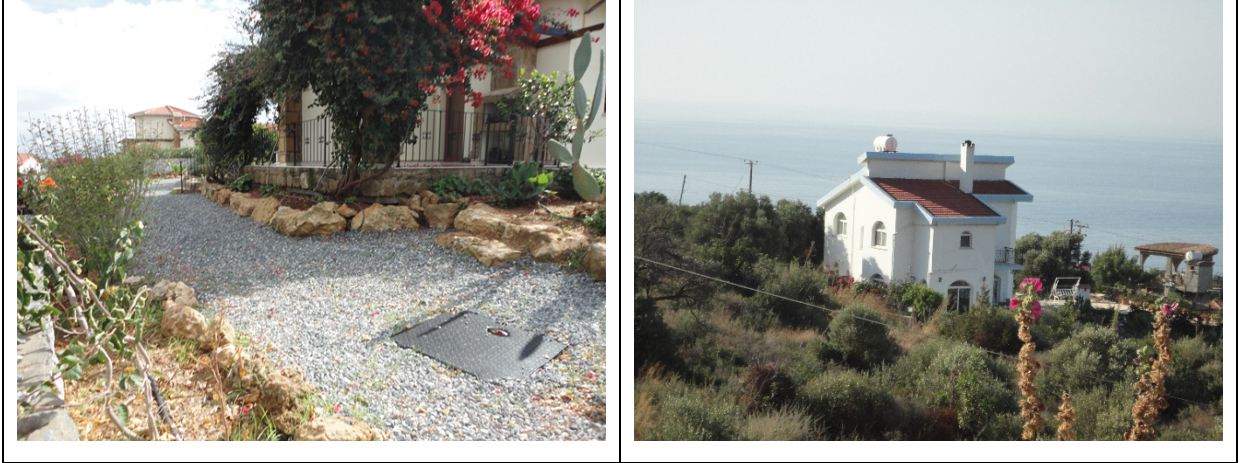
Figure 6. View from the new residential region
