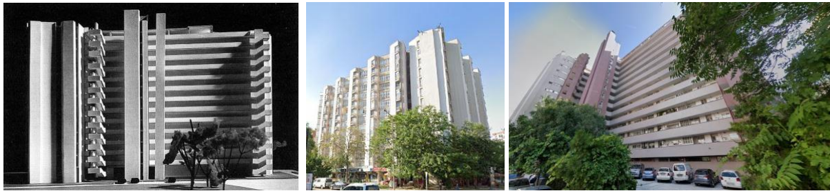
Figure 6. Yeşil Meram residence facade view (Url-4, 2024)
