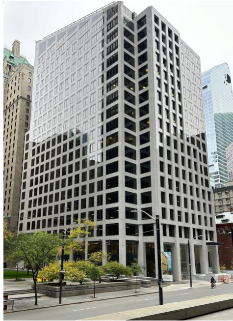
Figure 6. Revitalized 95 Wellington Street building with a ventilated facade having Bethel White Granite cladding, credit by: Steve Schrenk.
