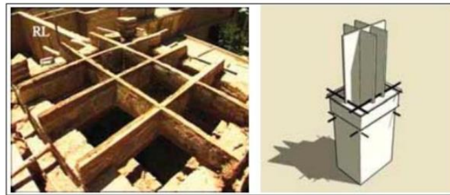
Figure 1. Sections of the Wind Tower (Farahza & Khajehrezaei, 2011)
