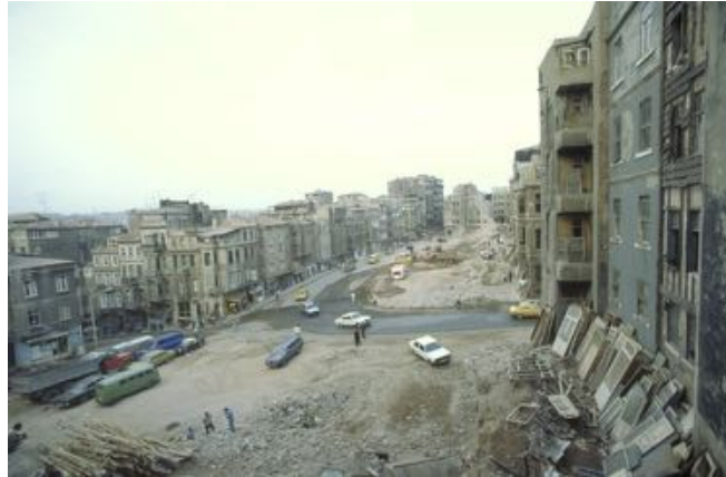
Photo 13. Demolition Works for the Opening of Tarlabası Boulevard https://twitter.com/hayalleme/status/1141602834426814464/photo/1
