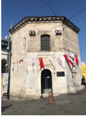
Photo 2. Istanbul Metropolitan Municipality Information Center (October 2022)
