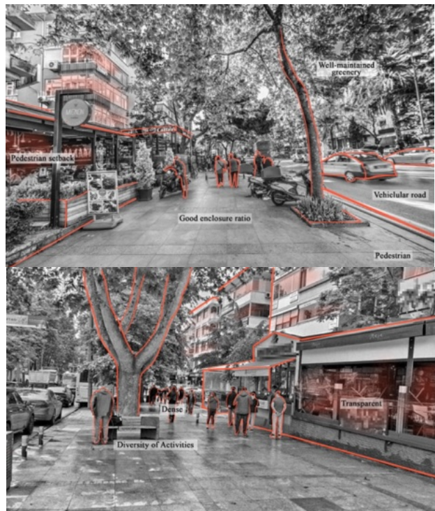
Figure 3. Photos taken from the active street interface type at Bagdat Avenue/ Kadikoy.
