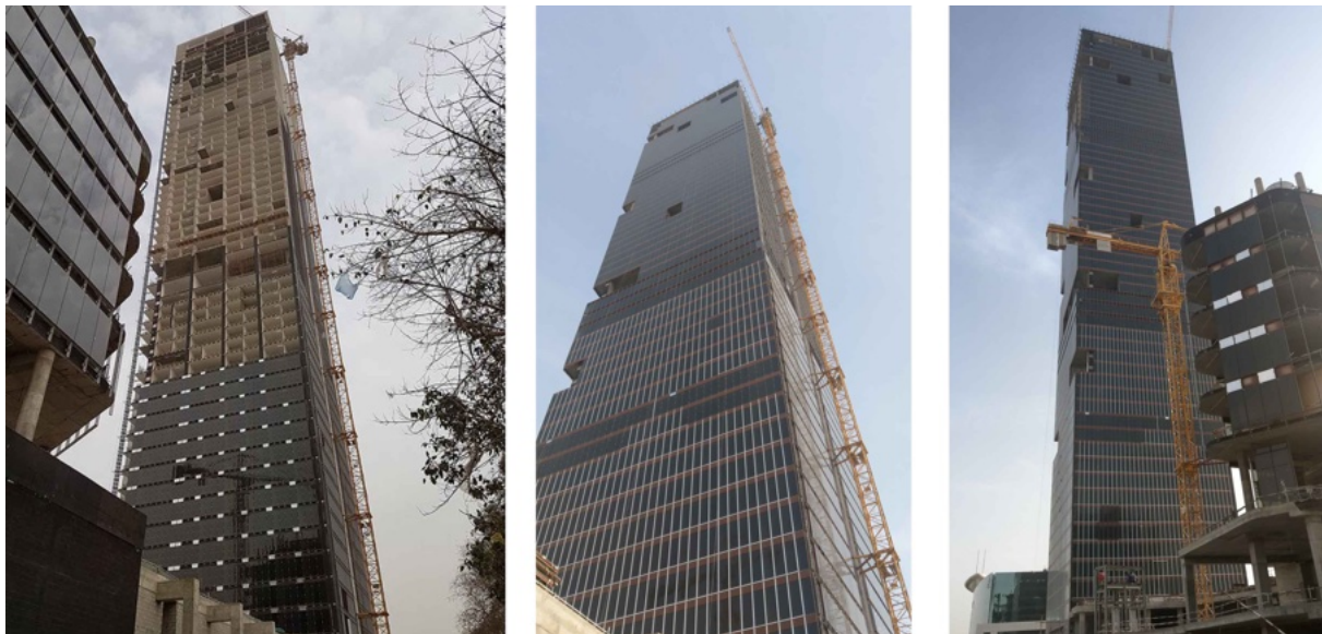
Image 8: Pictures captured during the construction phase of project (Skycity, 2020).
